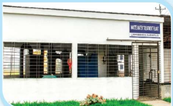
Waste Water Treatment Plant
