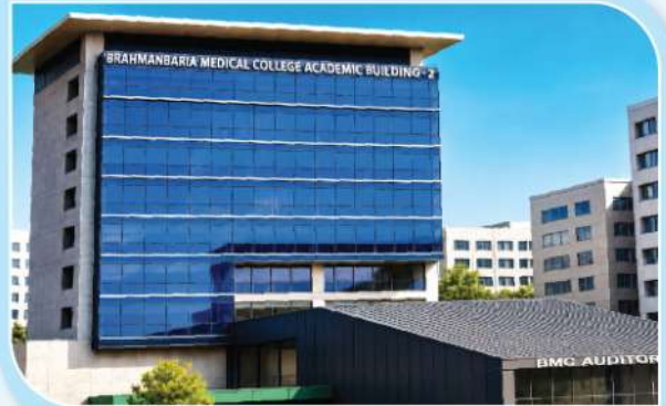
Under Construction Academic Building : 2
